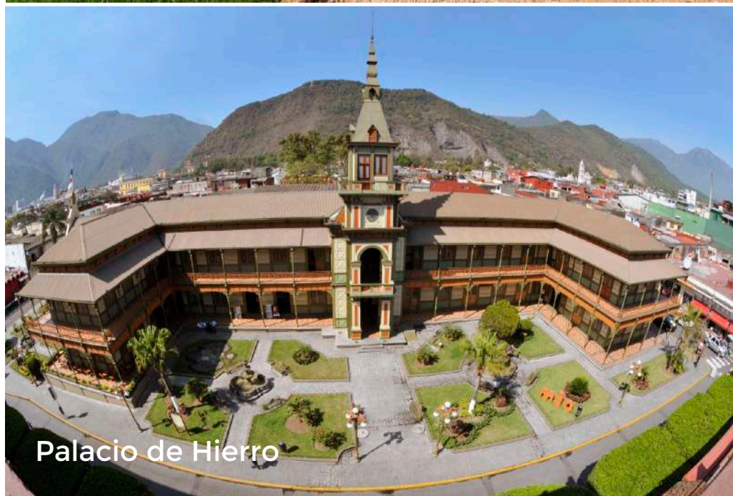
Rio Blanco Former Textil Factory
